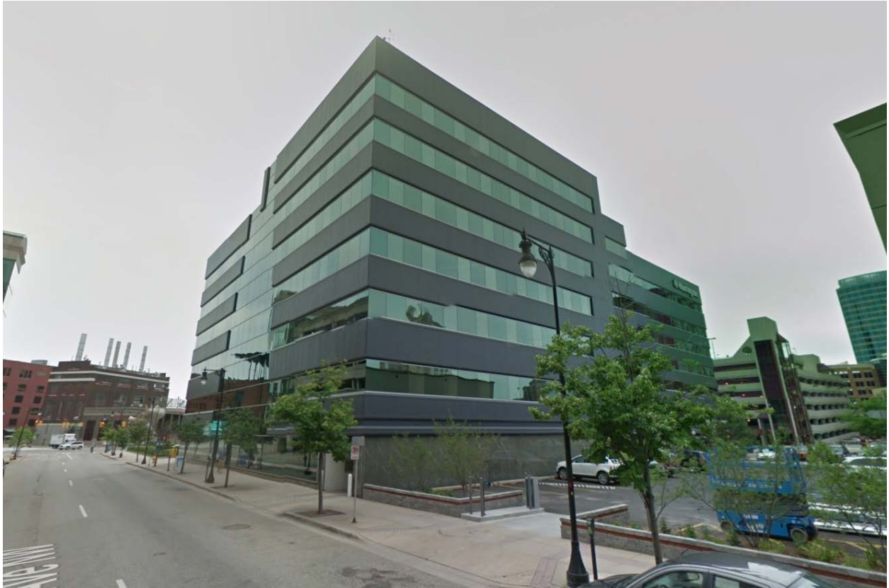
Existing Ottawa Ave frontage (NE elevation)
